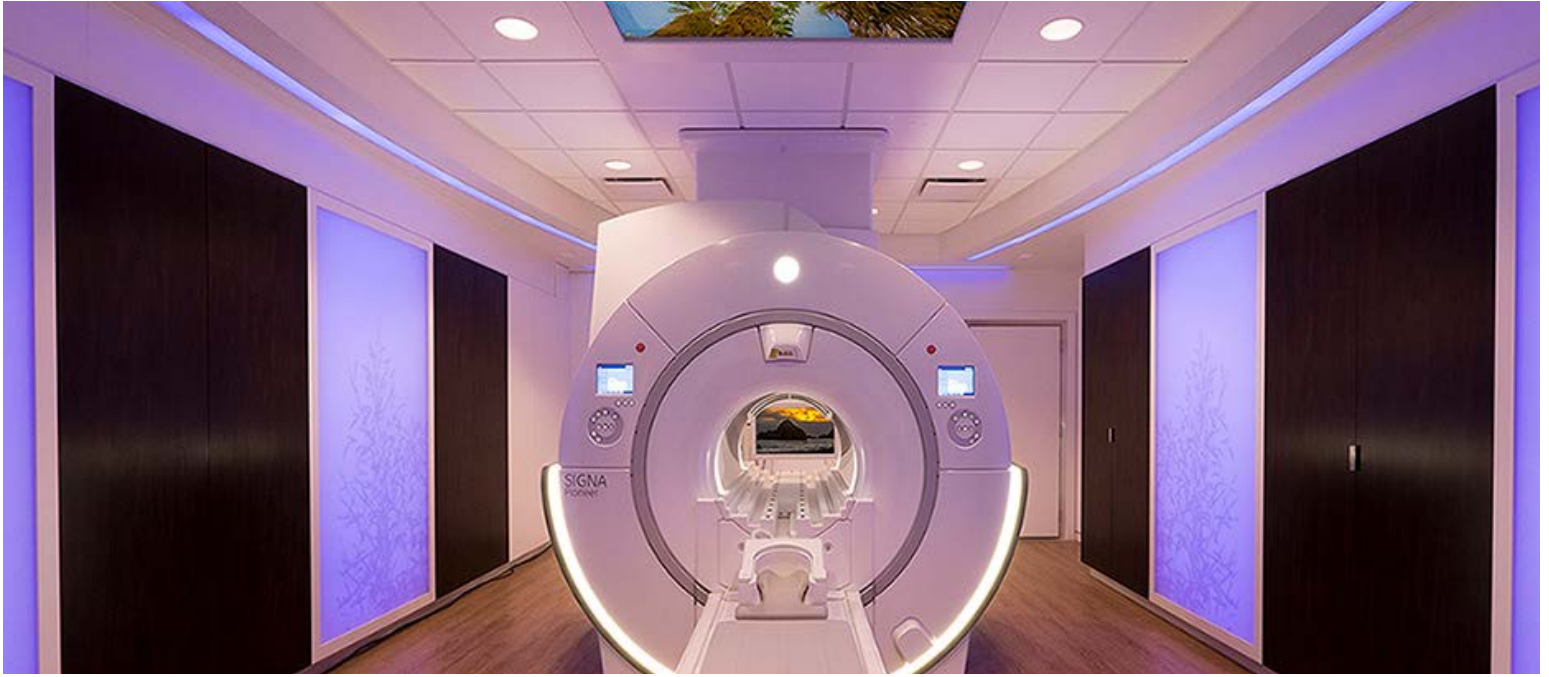
Head-First Scan - MRI Wireless Video Display is placed behind the bore. Patient uses mirror glasses, head-coil mirror or bridge mirror to see display
